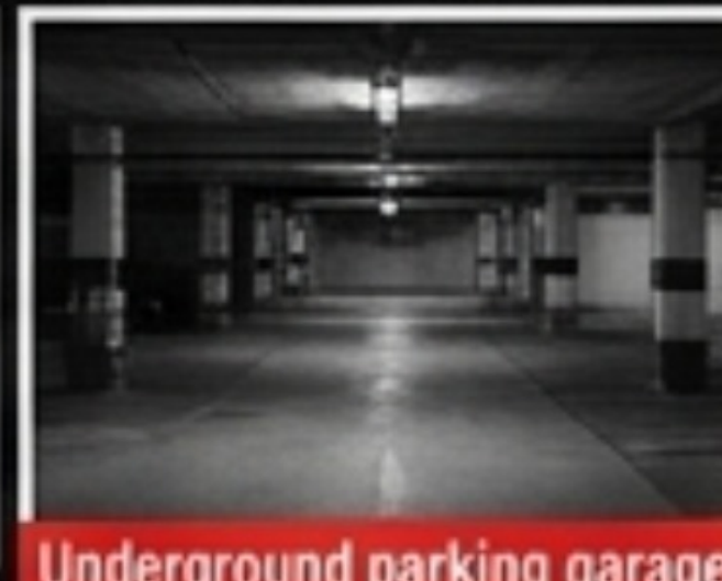
Underground parking garage
